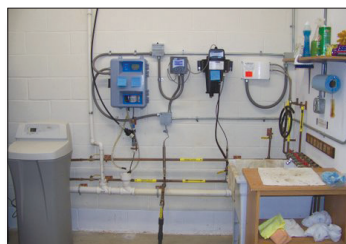
Inline turbidimeter and chlorine residual analyzer
