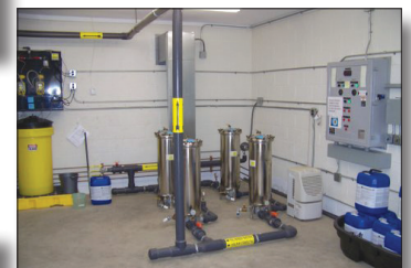
Cartridge filters and hypochlorite system
