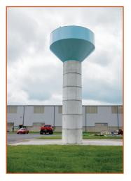
which resulted in a rapid response by industry leaders. Double ellipsoidal, radial cone and water spheres were commonplace in the 1930s and '40s, followed by spheroidal, hydropillars and, in the 1980s, the composite elevated tank. Capacities over the same time increased from 50,000 and 100,000 gallons to tanks as large as 4-million-gallon capacity.
