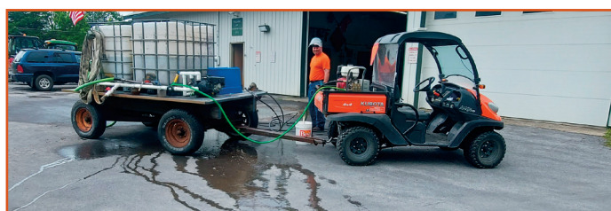
Water Wagon with paint removal system
