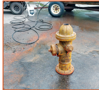
After old paint has been removed
