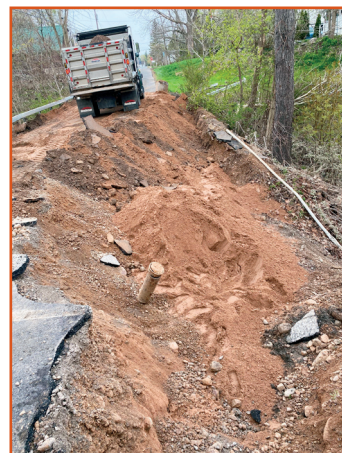
Repairing Road with fill
