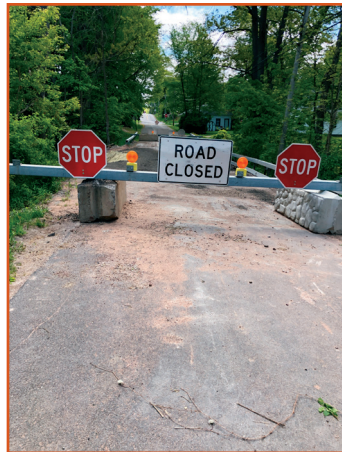
Bridge St. temporary road repair
