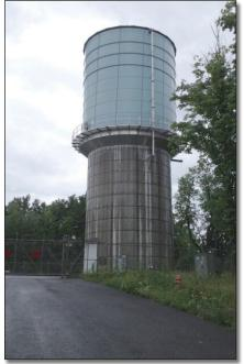
This tank is located in the Town of Brutus and is a 308,000 gallon elevated Aquastore tank. What was interesting about this location was the paved access road leading up to the tank easily cost more than the tank itself.
