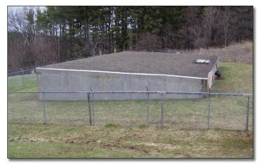
The next tank was a Sealstore Tank (early 80's) about 120,000 gallons located in the Hamlet of Erieville, NY. This tank served the district well until 2013 when corrosion finally took its toll on this early design. The second photo shows the operator's attempts at plugging the leaks by sharpening pieces of nearby underbrush and pounding them into the holes. This tank was replaced by a new Aquastore tank in 2014.
