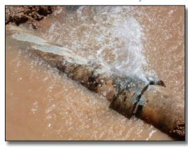
Checking the excavation, we determined that the as built was 30" off. How could that be? It was an as built therefore it was gospel. I guess not. The main was relocated putting a strain on our budget.
