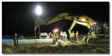
Backhoe lights are not enough to illuminate a night time work site and auxiliary lighting with a generator is a must.
